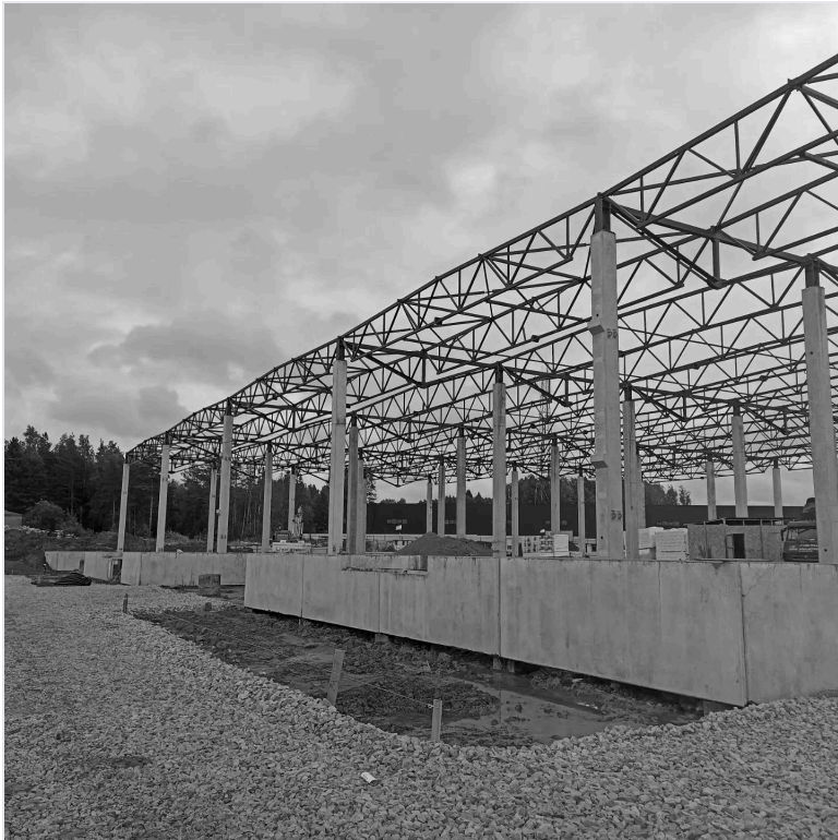
Fig. 31a–f — On-Site Construction Archive (KiPro Architectural Delivery): Precast concrete column erection, long-span steel roof truss assembly, insulated sandwich panel envelope mounting, and dock pit interfaces across 370,000 m 2 of logistics facilities.
