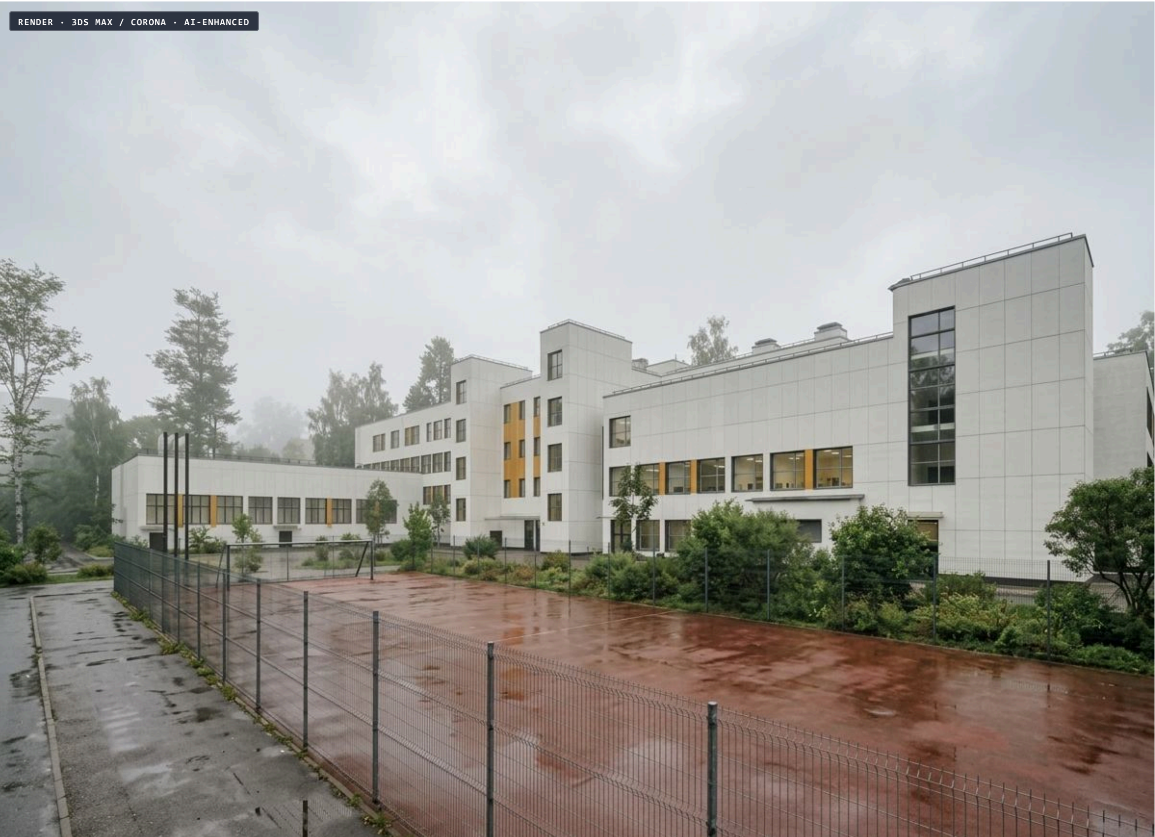
Fig. 05 — Courtyard and Outdoor Athletic Grounds: Ventilated rainscreen facade with accented window reveals, ribbon glazing, and sports grounds.
