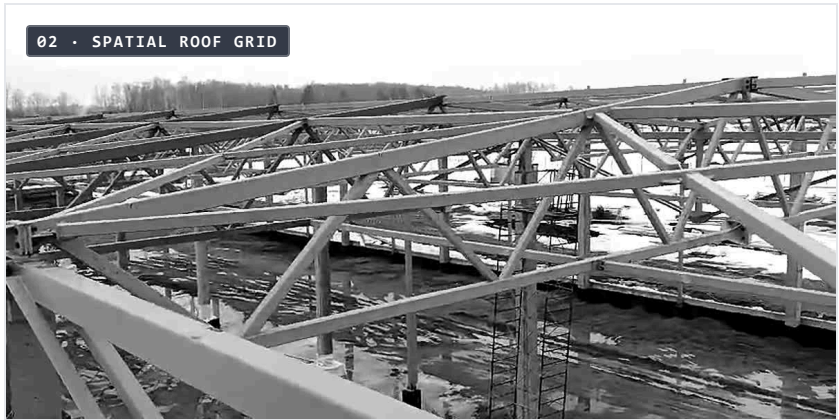
Fig. 27b–c — On-Site Structural Assembly (March 2024): 1) Mobile crane hoisting prefabricated steel roof trusses; 2) Spatial tubular steel truss structure across 132 m primary production bays.
