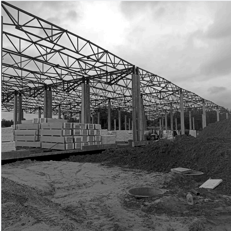
Fig. 31a–f — On-Site Construction Archive (KiPro Architectural Delivery): Precast concrete column erection, long-span steel roof truss assembly, insulated sandwich panel envelope mounting, and dock pit interfaces across 370,000 m 2 of logistics facilities.
