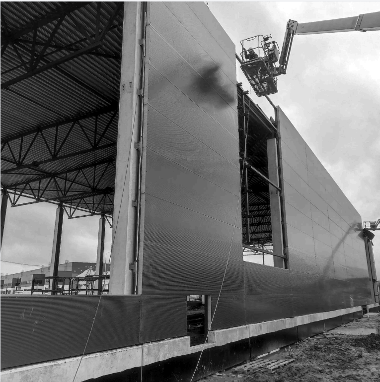
Fig. 31a–f — On-Site Construction Archive (KiPro Architectural Delivery): Precast concrete column erection, long-span steel roof truss assembly, insulated sandwich panel envelope mounting, and dock pit interfaces across 370,000 m 2 of logistics facilities.
